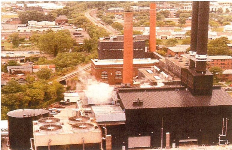
GPU International / Syracuse University Syracuse, New York 80 MW Cogeneration Plant
