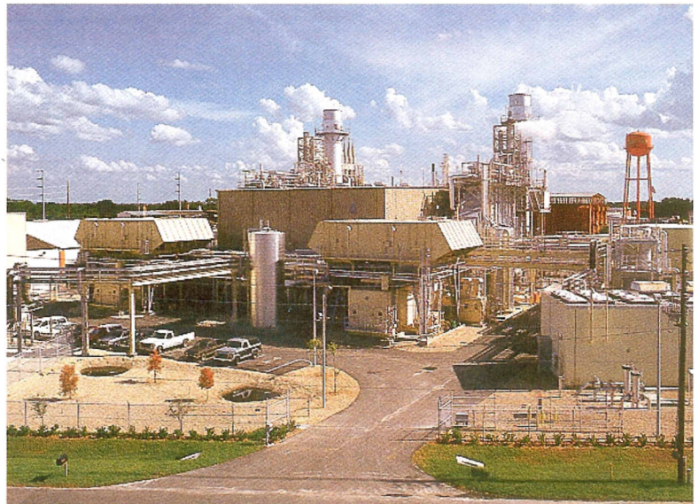
Peoples Gas / GPU International Umatilla, Florida 110 MW Cogeneration Plant
